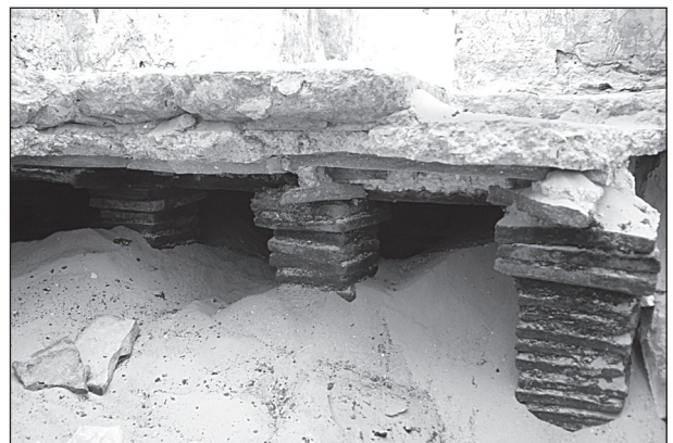
8. Cross-section of hypocaust in tepidarium (Th. Fournet).
