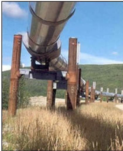
**Figure 2.1- Elevated section of Trans Alaska Pipeline [2]**
