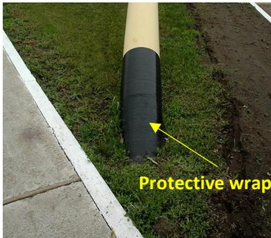
**Figure 2.10 – Protective Wrap on Pipeline [56]**
