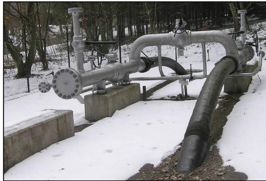
**Figure 2.9 - PIGs launcher and receiver station. [30]**
