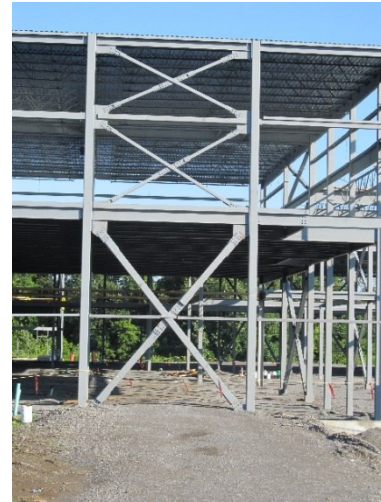
Figure 1.2. a) an MT-CBF in a sports facility; b) a two-tiered CBF in a single-storey shopping centre; c) a four-tiered CBF in a single-storey industrial building; d) a two-tiered CBF in the second storey of a two-storey commercial building.
