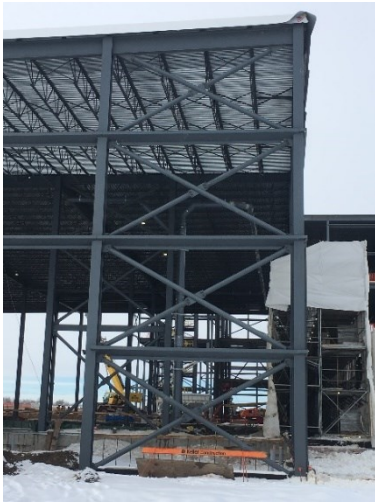
Figure 1.2. a) an MT-CBF in a sports facility; b) a two-tiered CBF in a single-storey shopping centre; c) a four-tiered CBF in a single-storey industrial building; d) a two-tiered CBF in the second storey of a two-storey commercial building.
