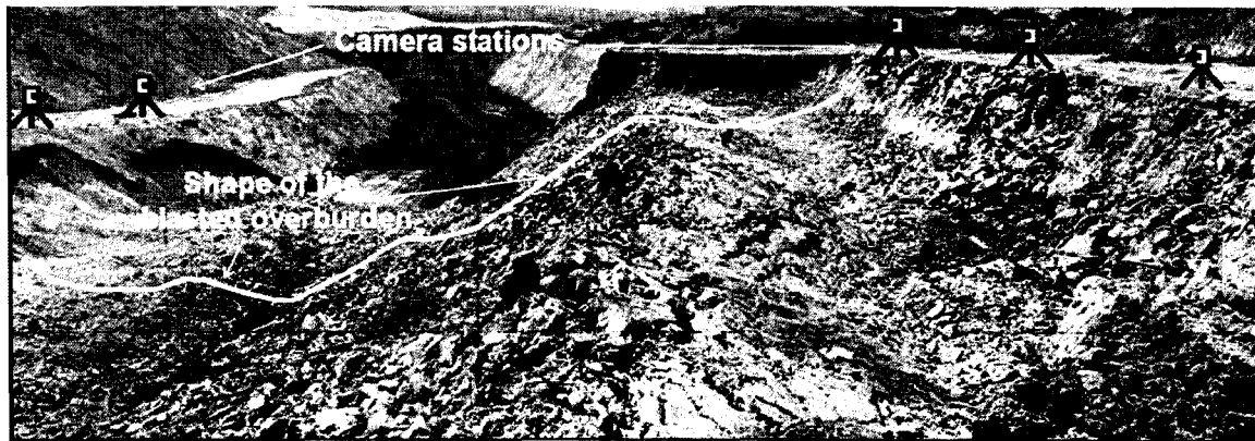
Figure 14 Shape of the overburden muckpile
