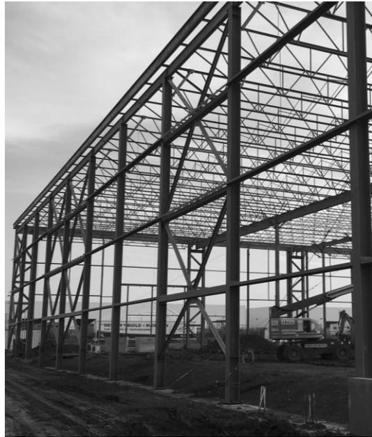
**Figure 1.1:** a) *four-tiered concentrically braced frame in an industrial building; b) two-tiered concentrically braced frame in an industrial building.*
