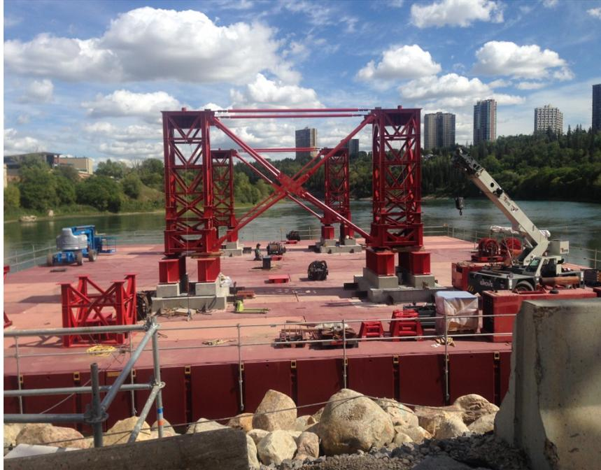
Figure A-3: Temporary Modular Barge (August 20<sup>th</sup>, 2015)
