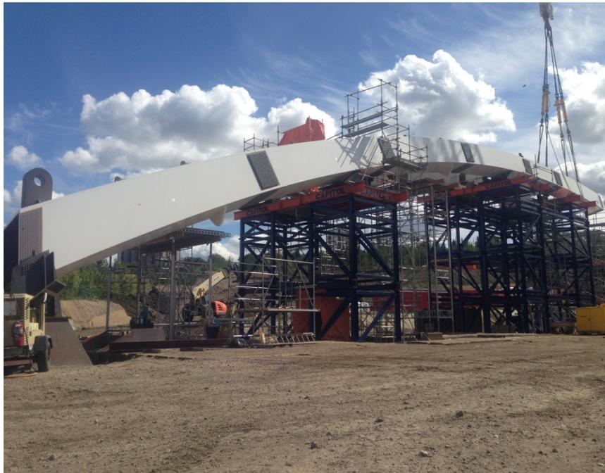
Figure A-4: Mid-arch Section Construction (August 20<sup>th</sup>, 2015)
