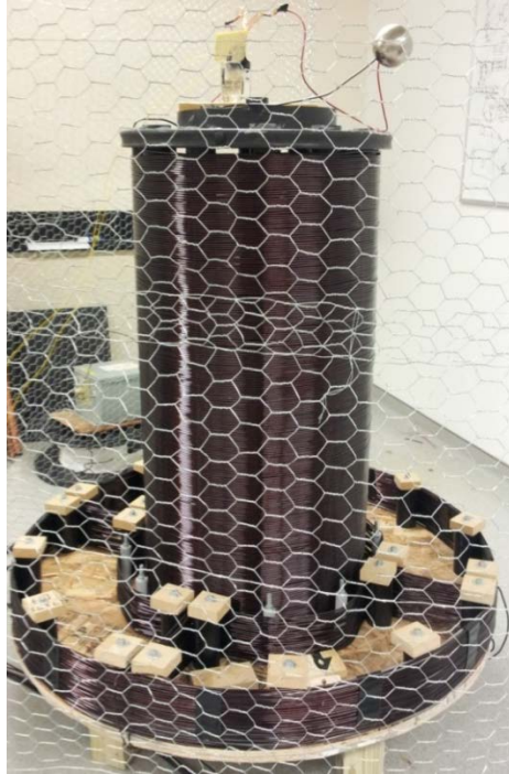
Figure 3-2 Near-field Resonant Auto-Transformer (NRAT) encased in Faraday's safety cage
