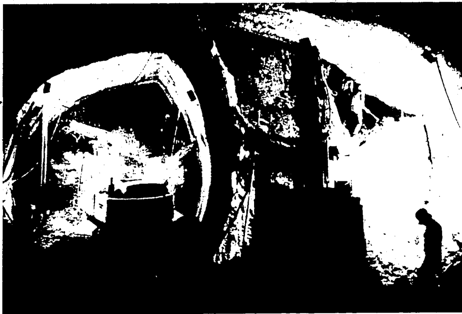
Plate 3.3 Tunnel excavation using scheme T3 (both photos reproduced from 'U-Bahn Linie 8.1', with permission of the U-Bahn Referat - München)
