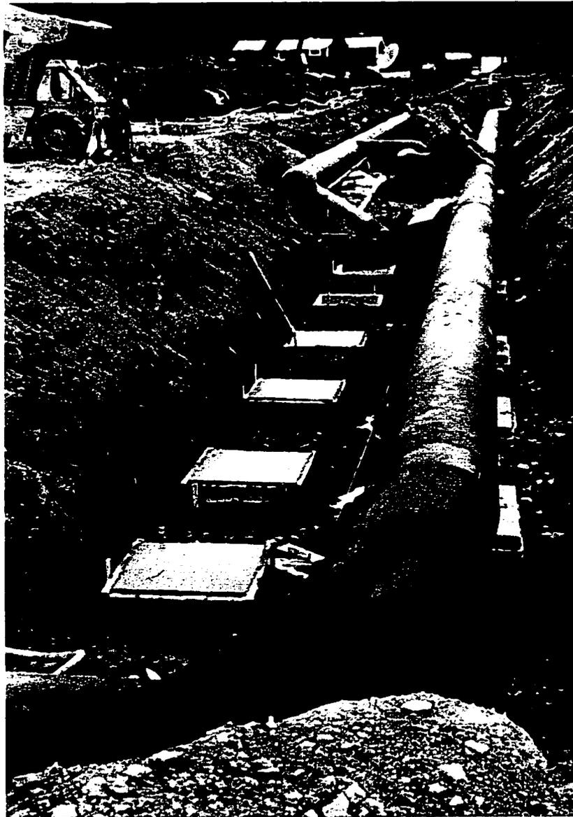
**Figure 1.1** Typical sleeper-supported pipe installation
