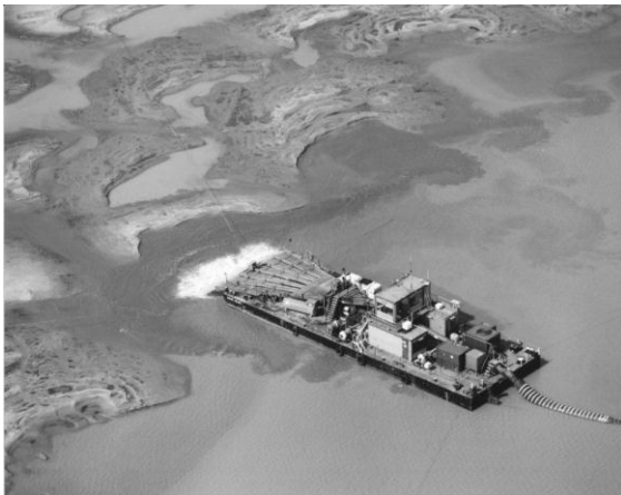
Figure 6. Computer-controlled spreader pontoon in shallow water. The sand-water mixture is distributed by a 12-m wide chute.
