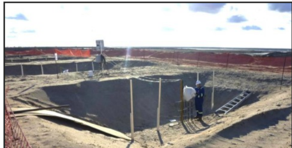
Figure 2. Cell 4 Before Filling.
