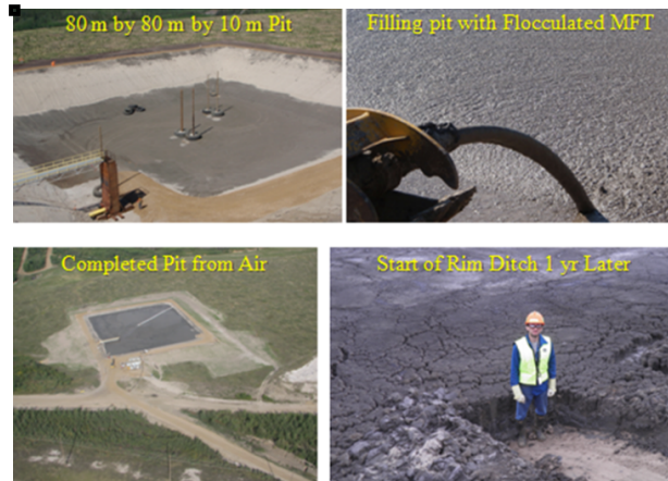
Figure 3. Syncrude 2009 Accelerated Dewatering Pilot.
