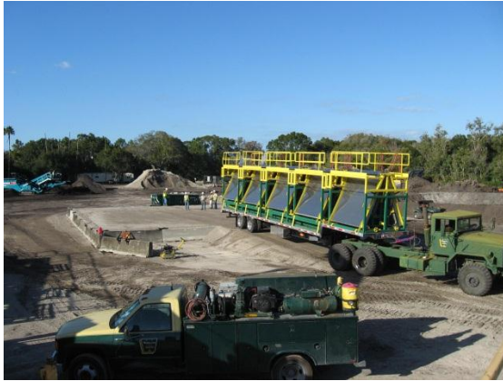
Figure 8. An AquaScreen Arriving at Site for Set Up.
