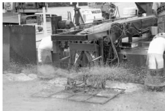
Figure 7. Detailed view of the sand capping process at the Fox River, showing a conveyor belt (right upper part) providing dry sand to a spreader device (middle).
