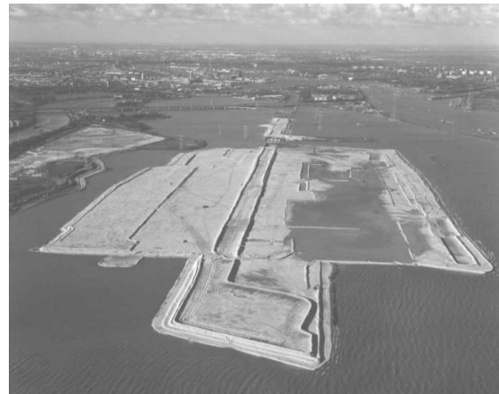
Figure 5. Overview of the IJburg Project showing the partly reclaimed area consisting of a layer of sand on top of a soft subsoil.
