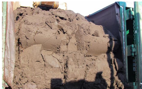
Figure 5. Solids Being Excavated from a TerraCore.
