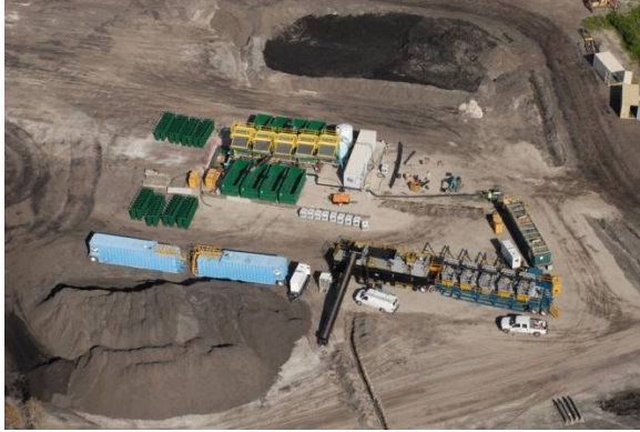
Figure 7. Equipment Set Up On Soil Washing Project.
