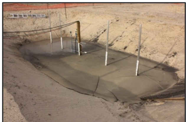
Figure 3. Cell 4, 21 h After Placing First Lift.
