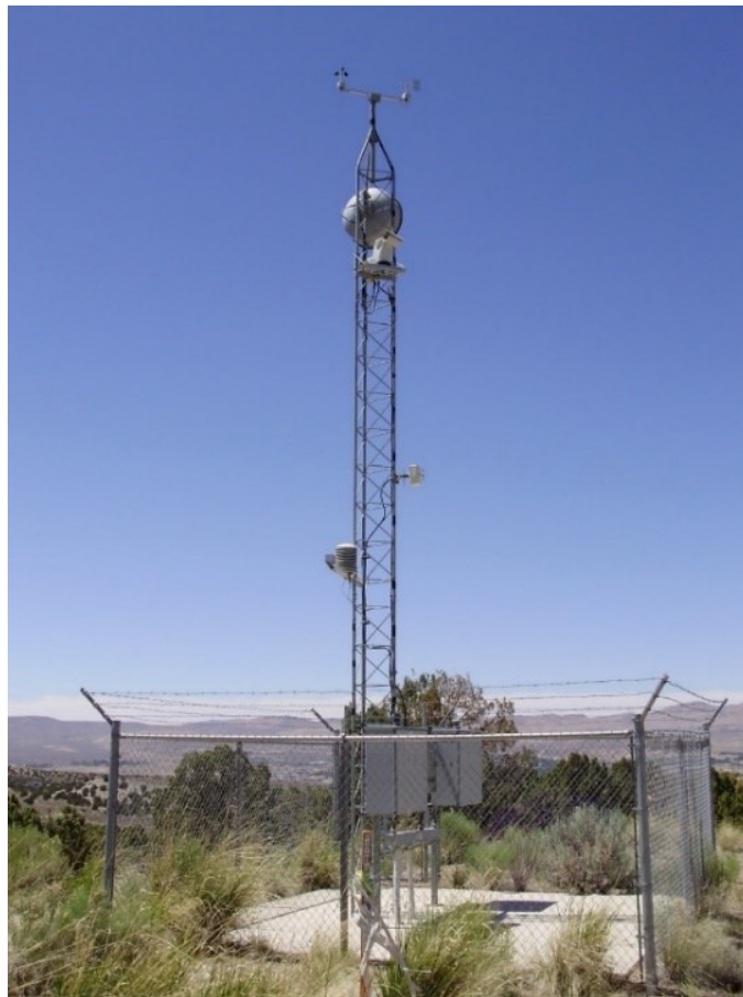
Figure 1-1 A typical stationary Road Weather Information Systems (RWIS) station
