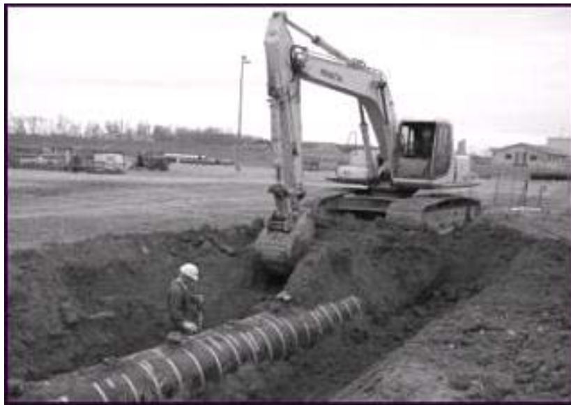
Figure 1.2 Excavation of a Pipeline
