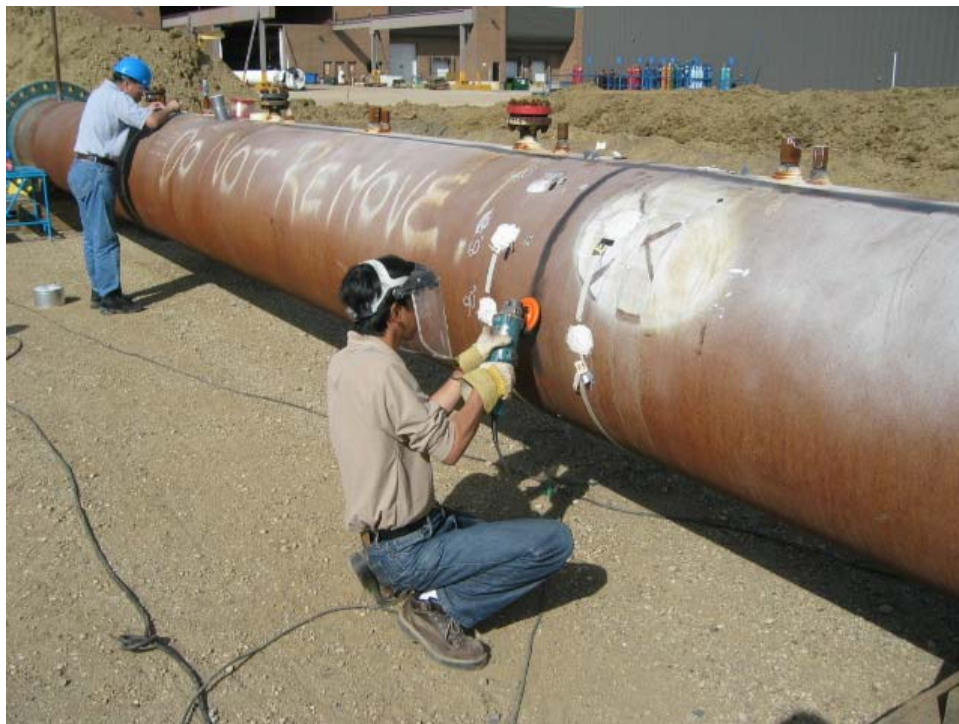
Figure 4.25 Surface Clean-up for the Field Line-Pipe
