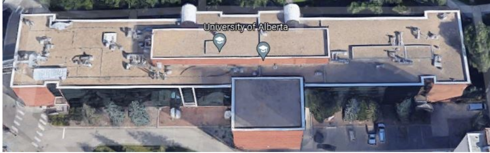
Figure 4. Google's 3D model of the EAS building. Imagery ©2021 Google, Imagery ©2021 Maxar Technologies, Map data ©2021
