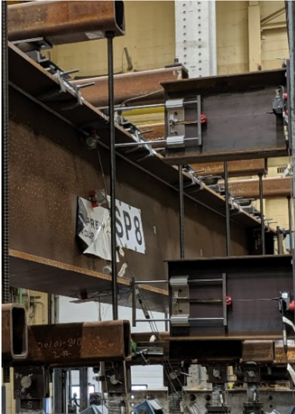
Figure 3-17: Miller-West Gliders showing differential flange displacements during buckling
