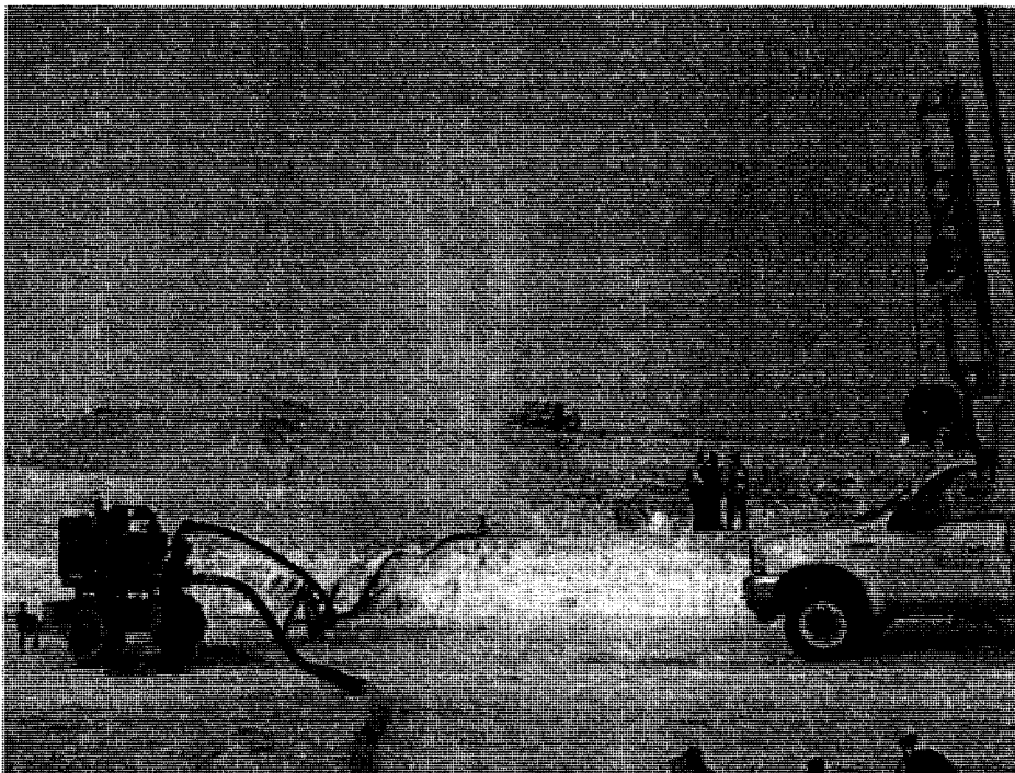
Figure A6.1 Spray Freeze Field Trial #2 – Hose, Pump and Nozzle in Operation
