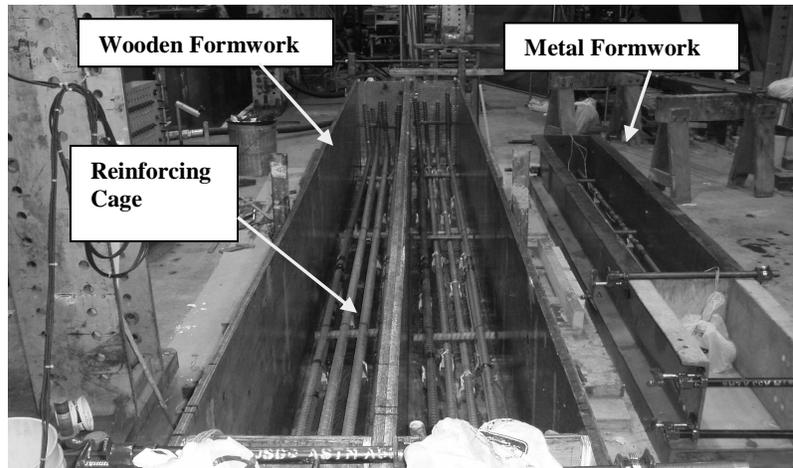
Figure 5-4: Formwork for specimens with  $h=308\text{ mm}$  &  $h=600\text{ mm}$
