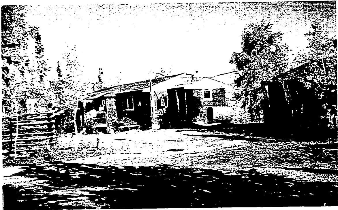
Figure 3-1. Discovery Mine Base Camp
