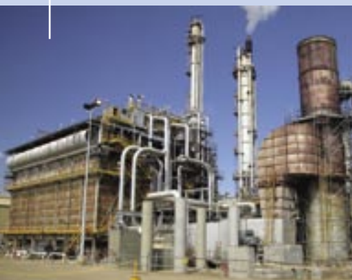
Syncrude uses natural gas to produce hydrogen, which is a key ingredient in our highly upgraded Syncrude Sweet Blend product. Shown here is the hydrogen plant at our Mildred Lake Upgrader.
