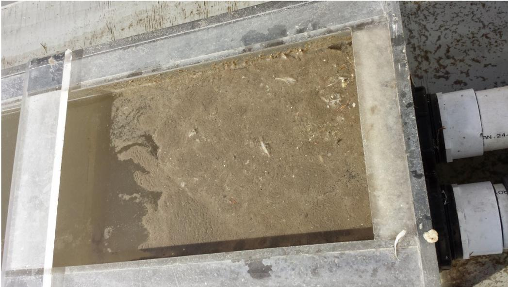
Fig. 39: Entrance section of the grit tank showing scum layer on the top of the water.
