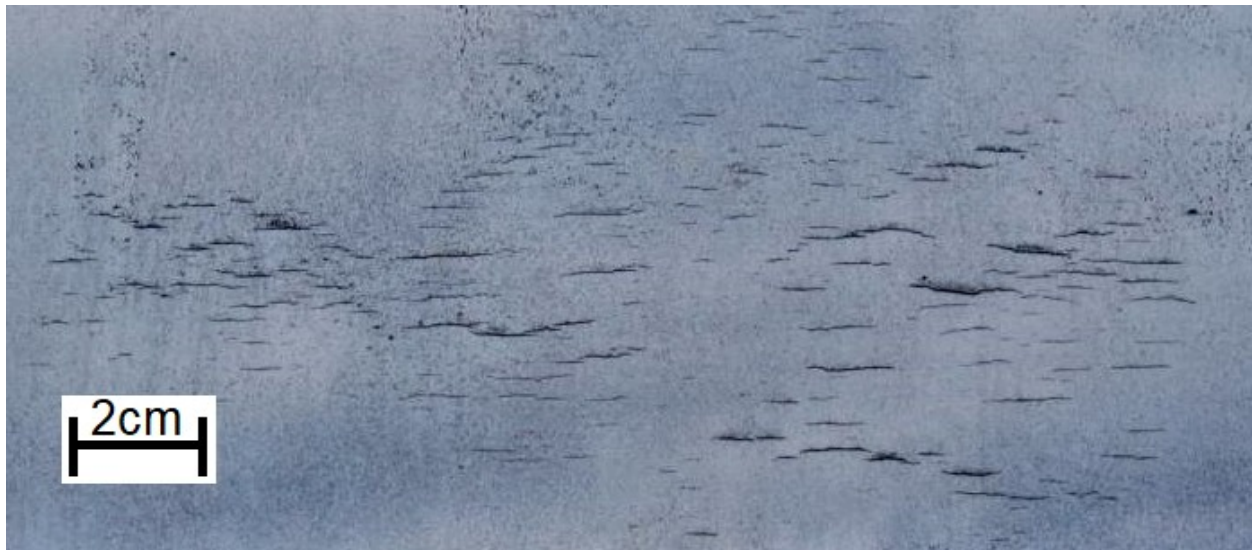
Figure 2.1. HpHSCC colonies on the external surface of the gas pipe detected by Magnetic Particle Inspection (MPI) [25].
