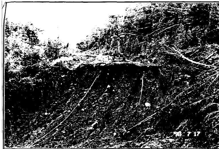
Figure 2-15 Earth slide at MP 150.10, looking south (Canadian Pacific Railway, photograph taken in July 1998)
