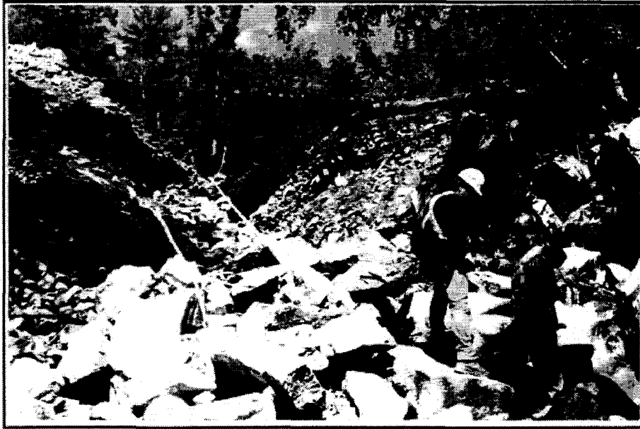
Figure A-3 Embankment erosion at MP 147.33 (Canadian Pacific Railway, picture taken in June 1998)
