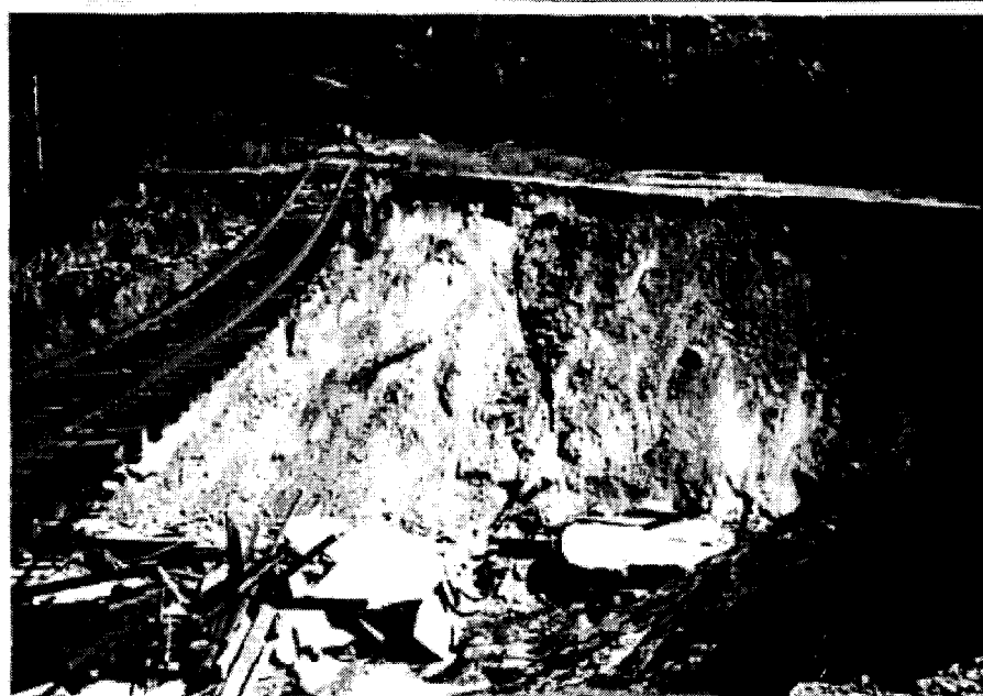
Figure 2-12 Embankment overland flow erosion at MP 154.47, looking south (Canadian Pacific Railway, photograph taken in June 1998)
