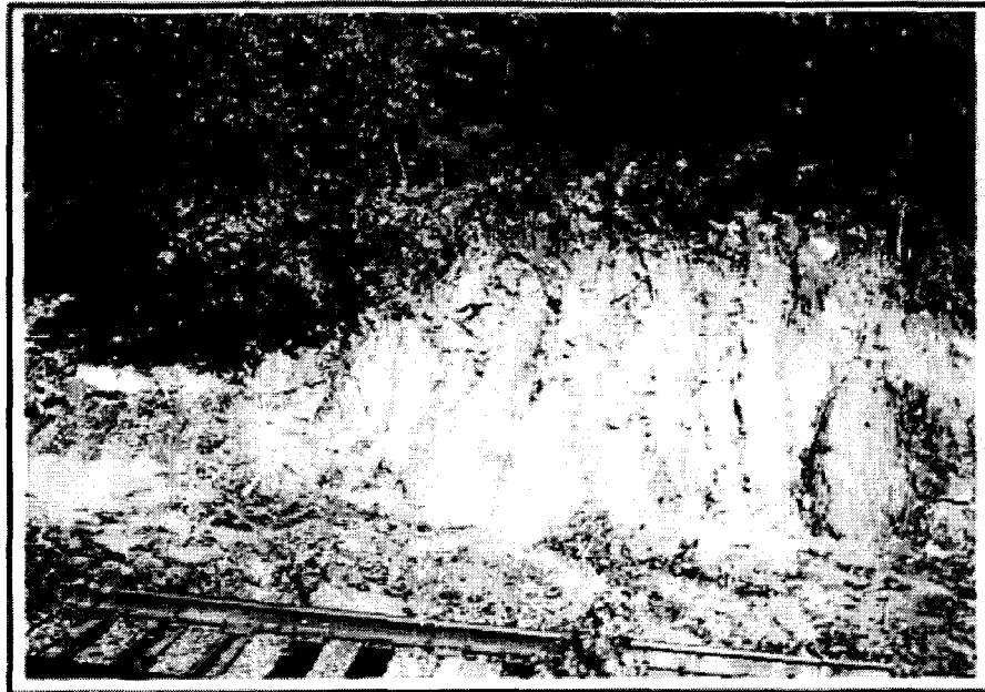
Figure 2-18 Upslope shallow earth slide at MP 151.30, looking west (Canadian Pacific Railway, photograph taken in July 1998)
