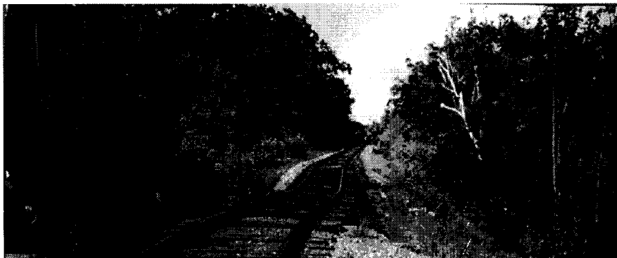
Figure 2-17 Embankment slide along railway (from Canadian Pacific Railway)
