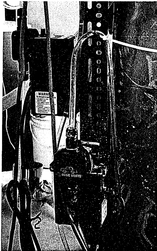
Figure 3-6 Chemical injection pumps
