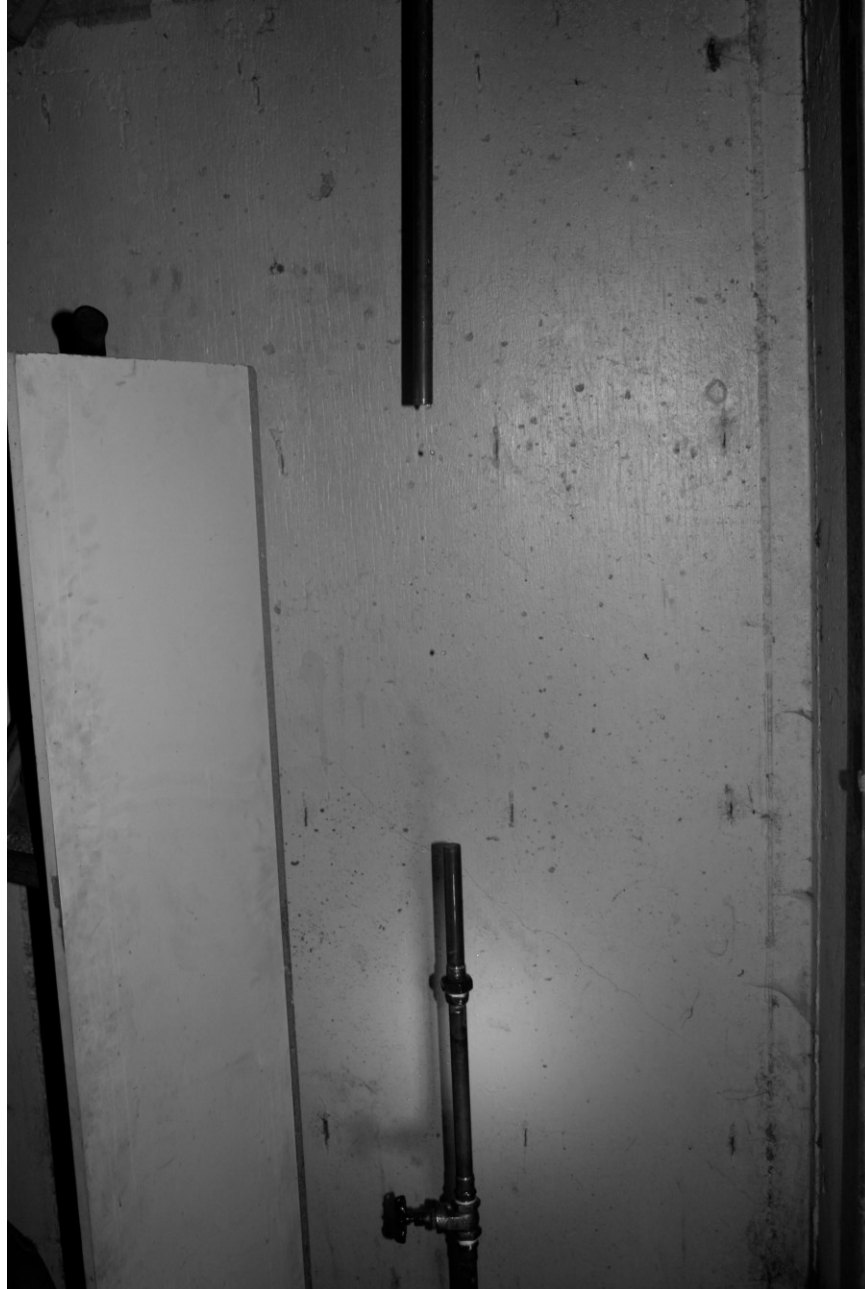
Figure 3.4 Water line section cut and removed above valve
