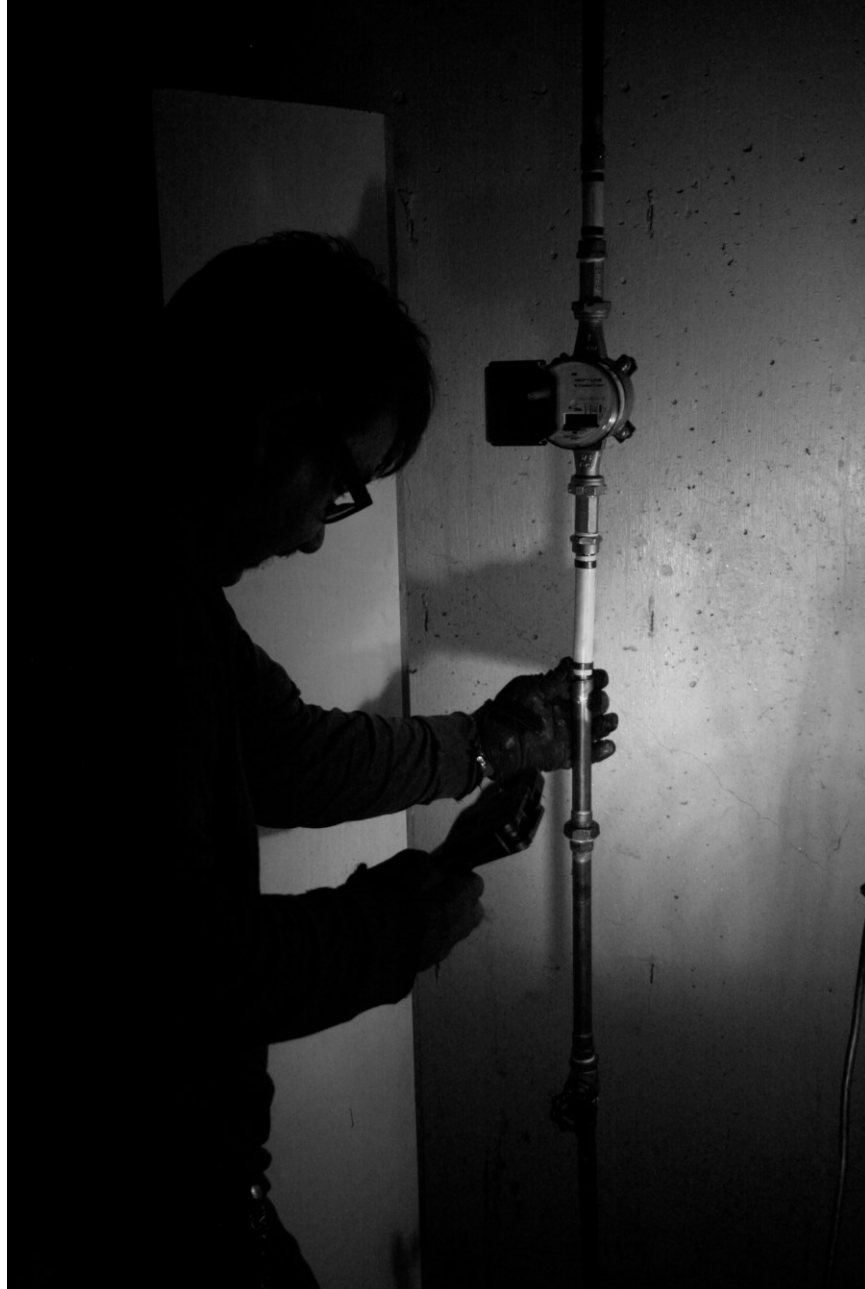
Figure 3.5 Plumber attaching water meter to water line
