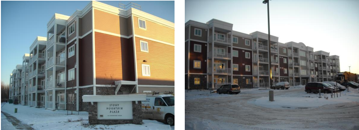
Figure 13: Selected case-study building
