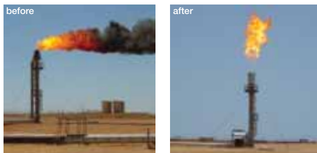
Enhancements to a flare stack at our central processing facility in Yemen have significantly reduced particulate emissions.
