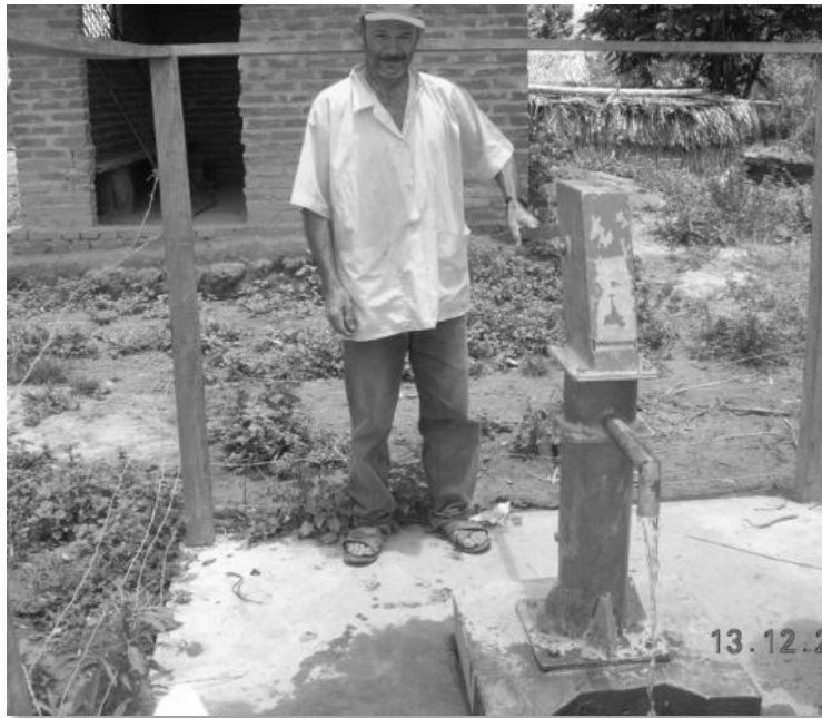
Figure 3-2 Principal manual water pump in Cerro Grande
