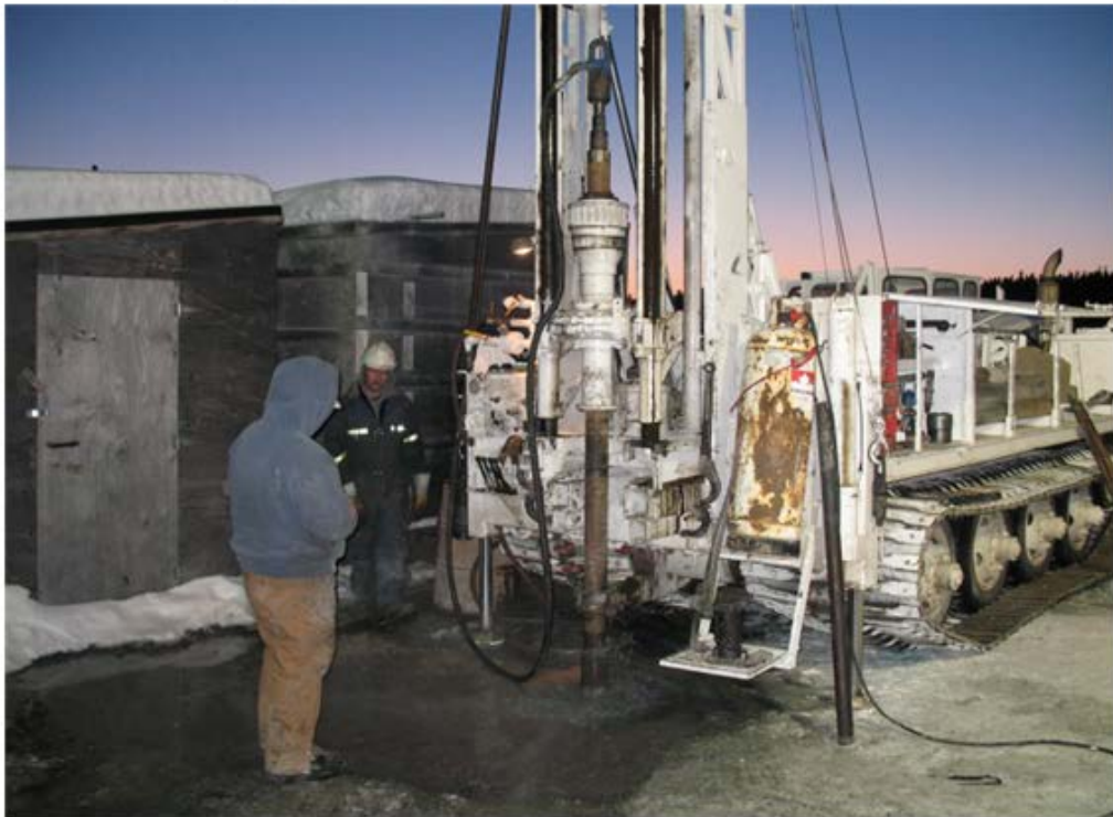
Figure E.3 Rotary percussion drilling machine used for coring and installation of new monitoring wells (MWs) in 2007 at the site.
