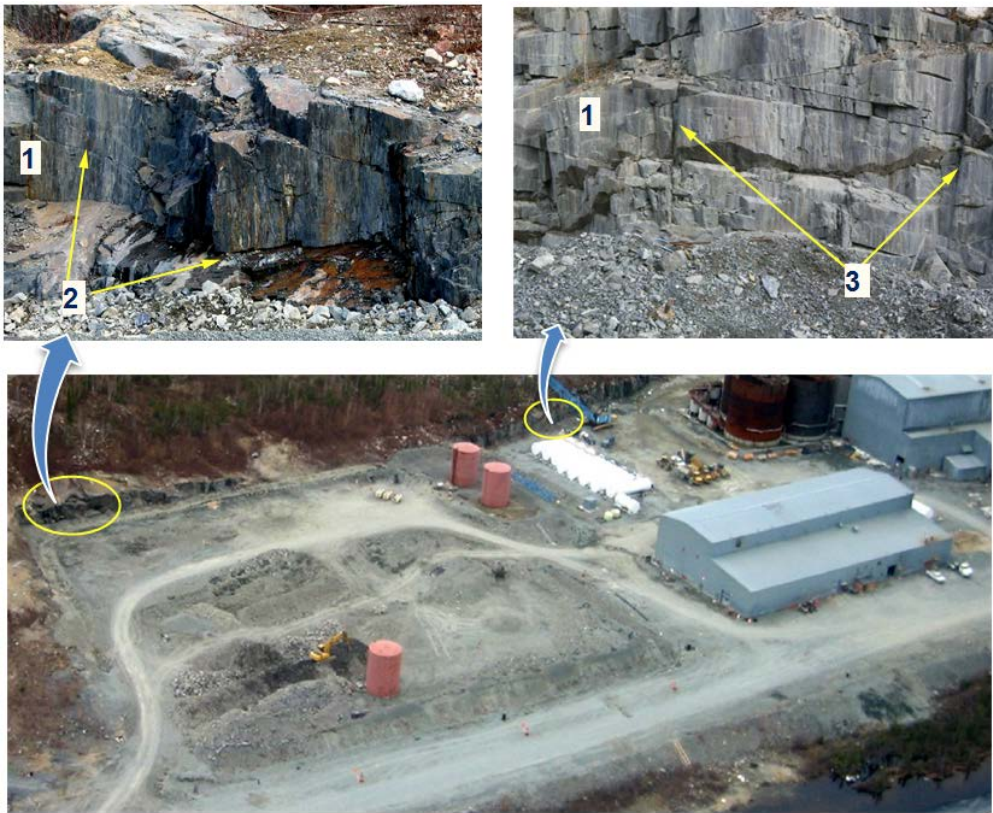
Figure H.2 Bedrock outcrop and escarpment showing (1) sub-vertical fractures parallel to foliation, (2) sub-horizontal fractures, and (3) sub vertical fractures parallel to 1 and 2.
