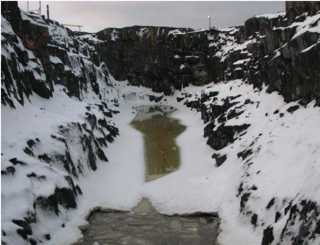
Figure H.8 Northwest view of the recovery trench showing free product accumulation on ice (modified after JWA, 2009b).
