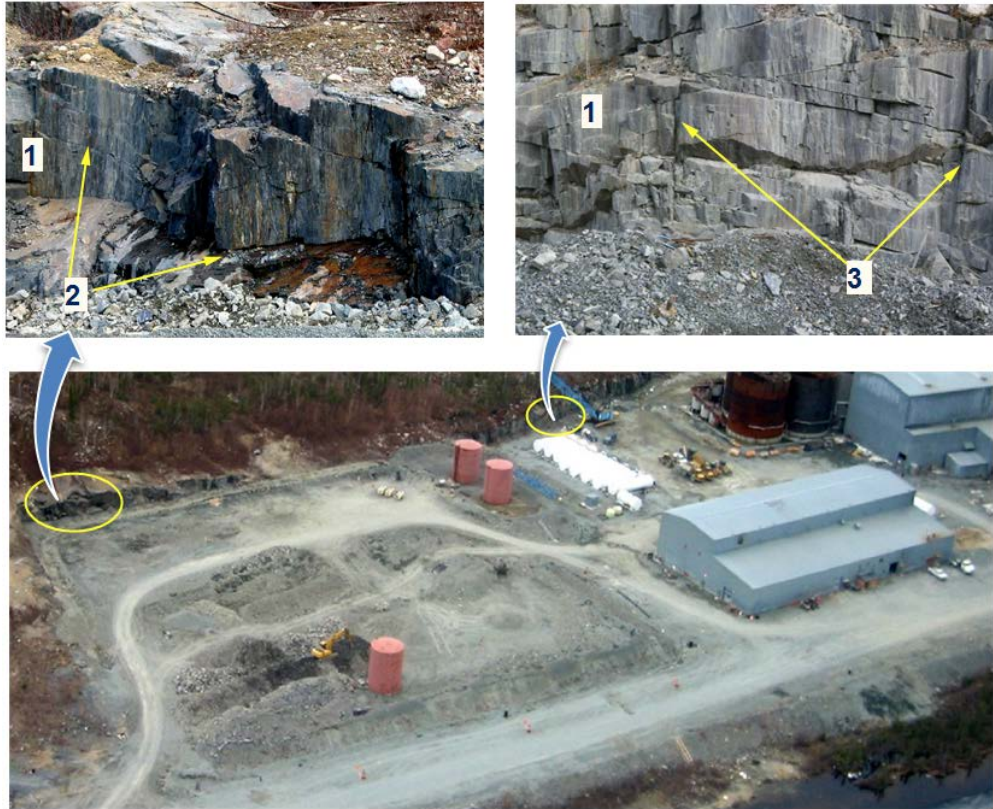
Figure 2.2 North to south trending bedrock outcrop with 3 main sets of fractures: (1) sub vertical fractures, parallel to foliation that includes “slaty cleavage” – includes most of the exposed surfaces shown in this picture; (2) sub-horizontal fractures; (3) sub-vertical fractures that are approximately perpendicular to 1&2.
