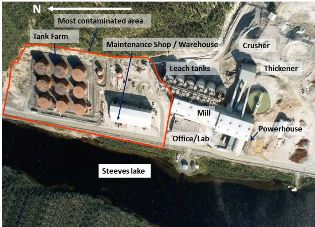
Figure 1.3 Layout of the mine site before demolition of the structures.
