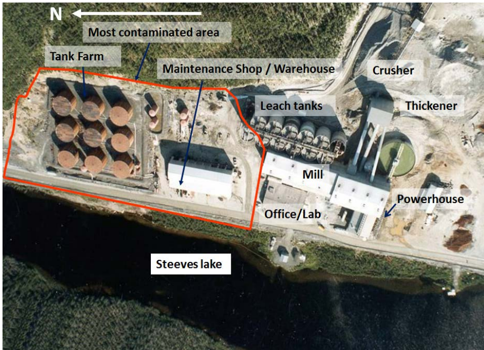
Figure H.1 Layout of the Colomac mine site before demolition of the structure during reclamation.
