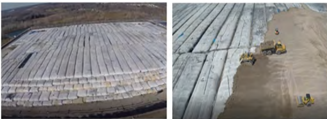
Photograph 4-17: Example of stacked geotextile tubes deposit including capping (adapted from TenCate Geosynthetic Americas).
