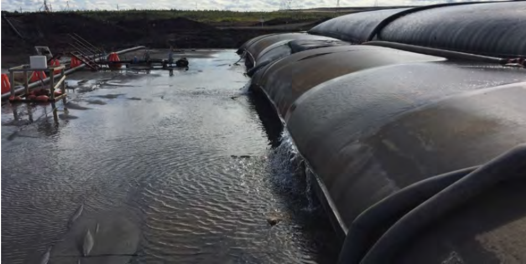
Photograph 4-13: Geotextile tubes field trial filling and dewatering.
