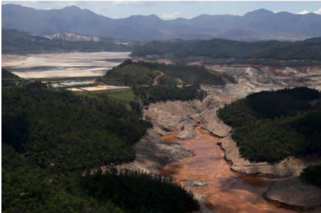
Photograph 5-2: Example of conventional tailings deposit flow liquefaction failure (Fundao – Brazil).
