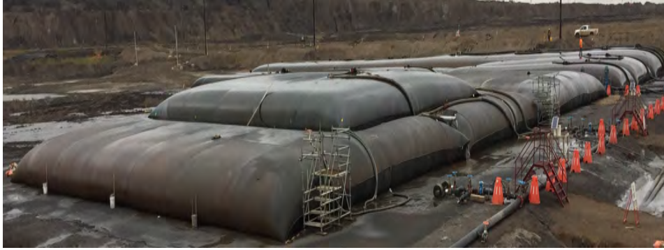
Photograph 4-16: Geotextile field trial completion of stacked 2 layers.
