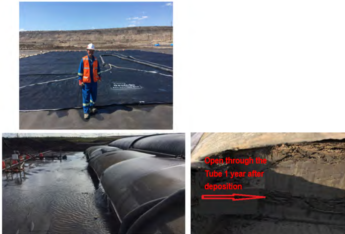
Photograph 1-2: Geotextile tube installation and accelerated dewatering and consolidation.
