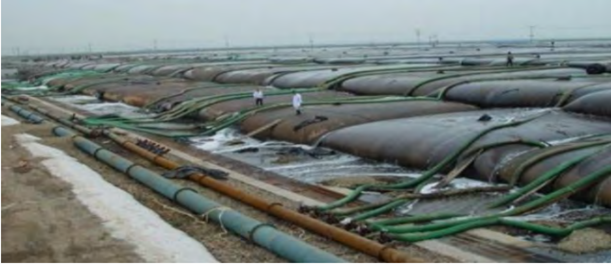
Photograph 5-3: Example of a large-scale application of geotextile tubes.
