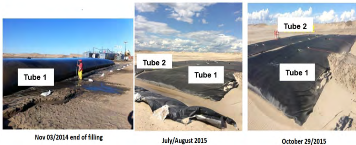
Photograph 4-9: Evaluating consolidation, dewatering solid contents and shear strength gain with time.
