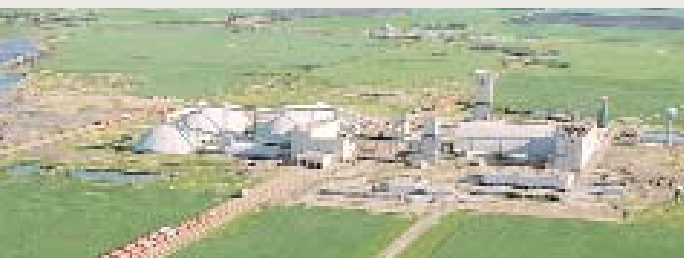
The Cory operation produces white muriate of potash products from conventionally mined potash ore.
