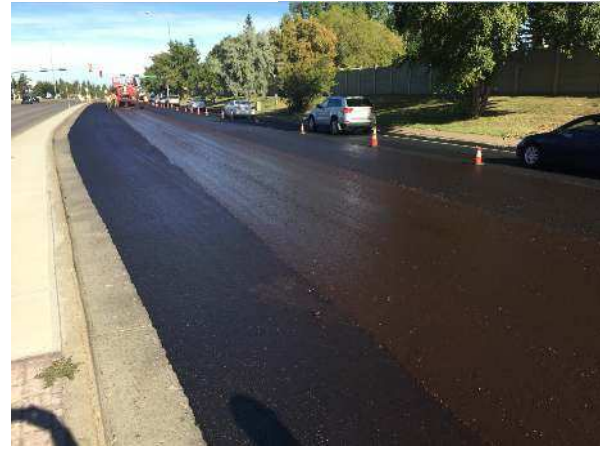
Figure 49A & 50B – Microsurfacing being applied on St. Albert Trail
