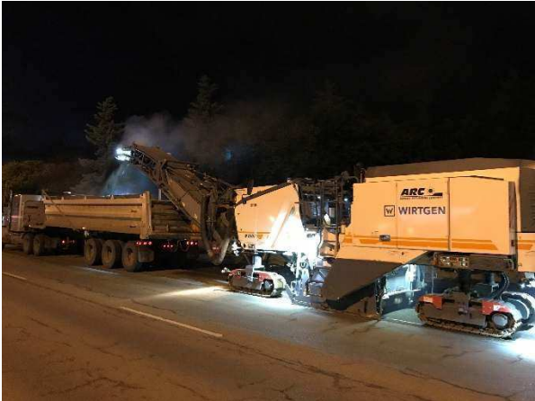
Figure 46a & 47b - Milling 50 mm depths
