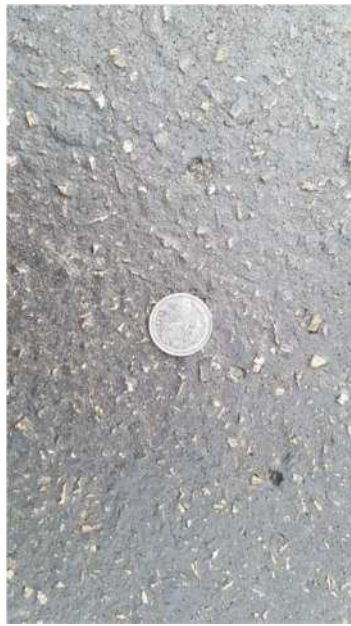
Figure 52a & 53b – (Left) SMA Surface Following Construction, (Right) Microsurfacing Surface Following Construction [46]
