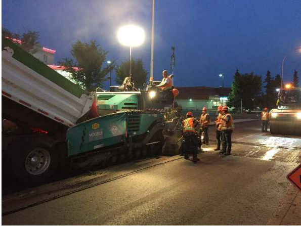
Figure 47a & 48b - Night Paving for SMA
