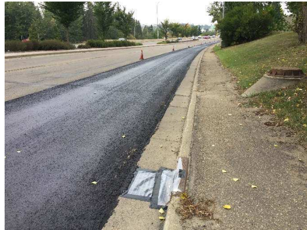
Figure 50a & 51b - Microsurfacing curing on St. Albert Trail
