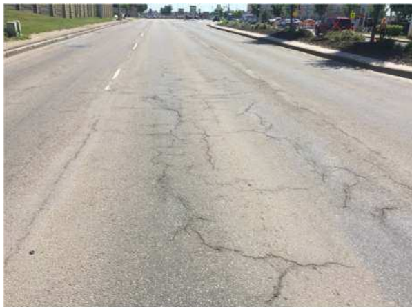
Figure 44A & 45B - (Right) St. Albert Trail near Grenier Place -HT Section, (Left) St. Albert Trail near Grenier Place (Microsurfacing Section)
