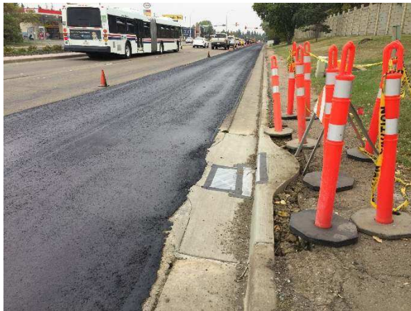
Figure 50a & 51b - Microsurfacing curing on St. Albert Trail
