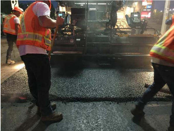
Figure 47a & 48b - Night Paving for SMA
