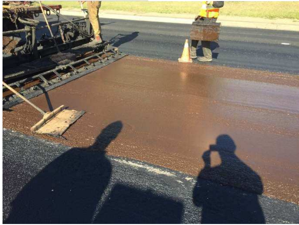
Figure 49A & 50B – Microsurfacing being applied on St. Albert Trail
