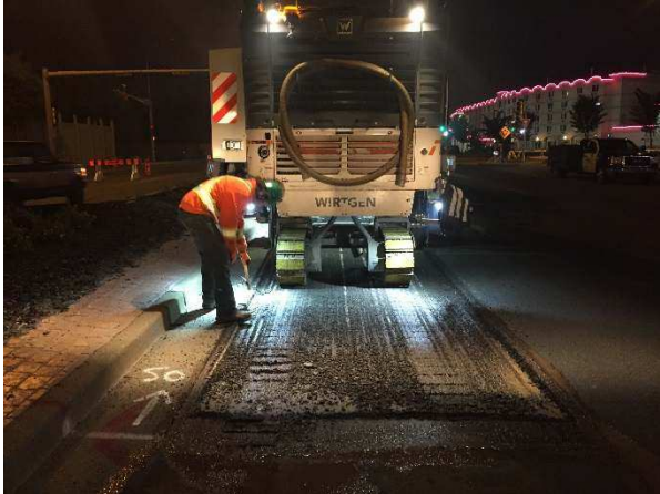
Figure 46a & 47b - Milling 50 mm depths
