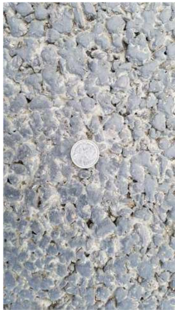
Figure 52a & 53b – (Left) SMA Surface Following Construction, (Right) Microsurfacing Surface Following Construction [46]
