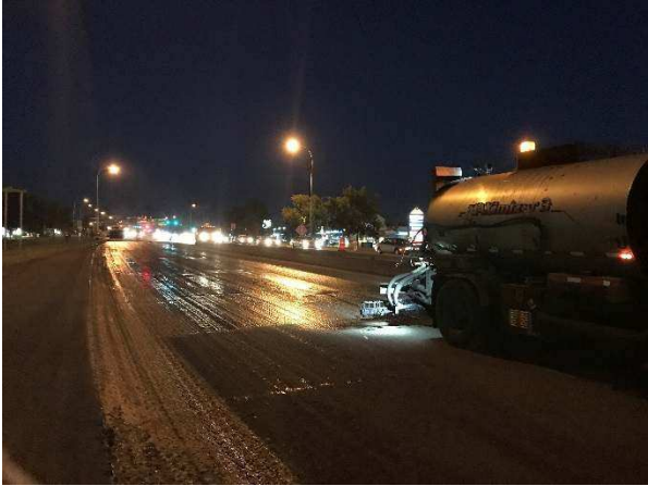
Figure 47a & 48b - Night Paving for SMA
