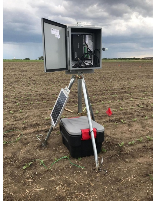
(b) Data logger, Multiplexer, Solar panel and Sensors.
