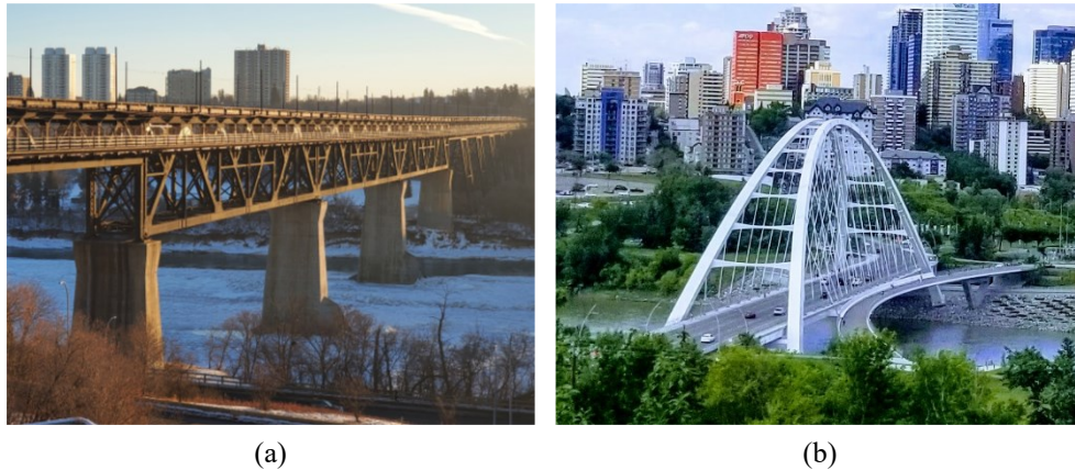
Figure 4-6: (a) The High Level Bridge and (b) the Walterdale Bridge that are considered in this study.
