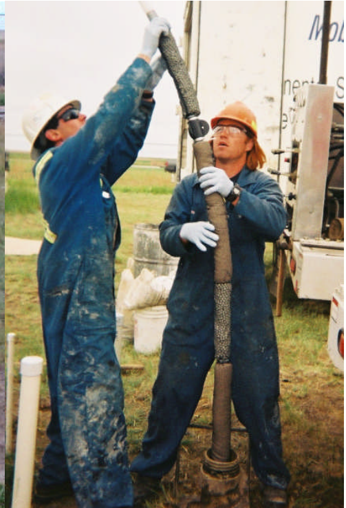
ML-well showing hand-sewn pre-pack frac-sand and bentonite pellet sleeves
