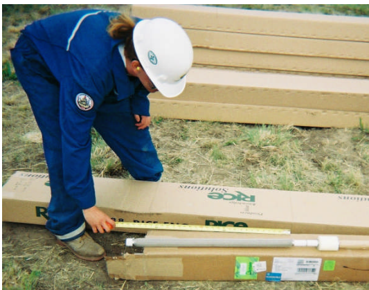
DP-pre-pack well screen, foam seal and paper wrapped bentonite seal to be placed inside driven steel pipe
