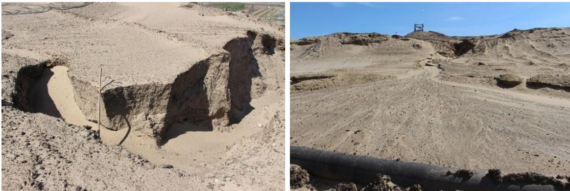
*Figure 6.5 Gully identified on north side of AOS tailings dam resulting from pooling water and concentrated flow (a, left), and resultant deposition of sediment in fan-like form (b, right).*
