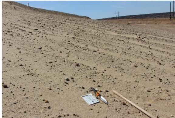
*Figure 6.6 Rills created by water erosion on north-east side of AOS tailings dam.*
