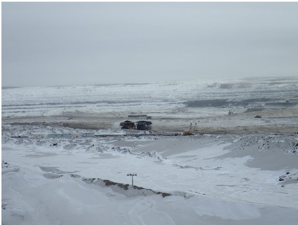
Winter Photo (a), Table 8. View of the open pit. Steep slopes ( \sim 55^\circ ) typical of mining operations and snow-covered benches.
