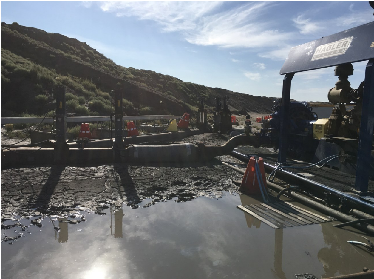
Summer Photo (d), Table 7. Pumps downslope of tailings dam. Pipes and associated structures in wet, soft ground conditions adjacent to slopes
