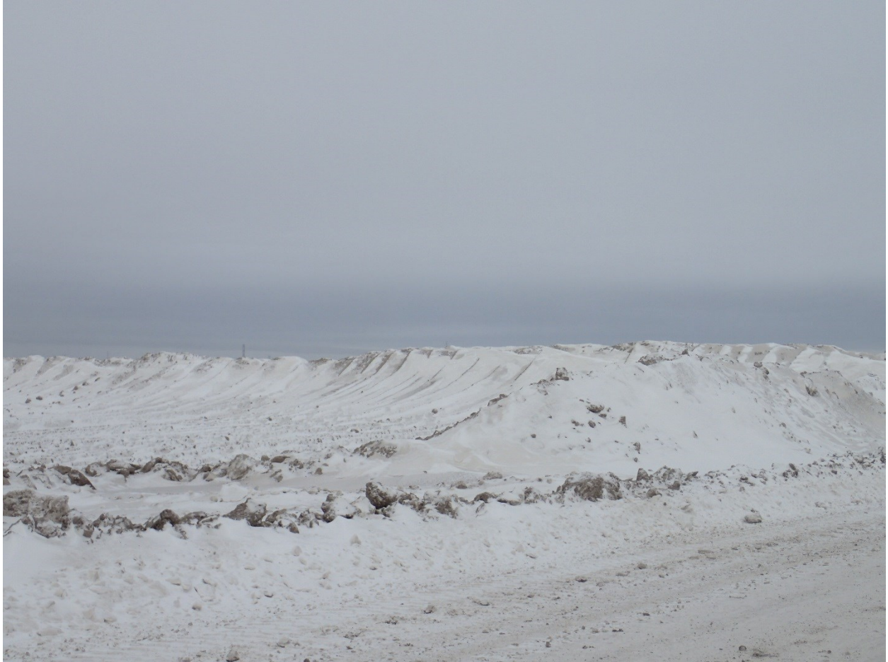
Winter Photo (b), Table 8. View of snow-covered eroded slopes of tailings dam.
