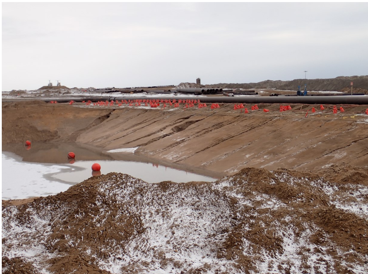
Spring Photo (b), Table 9. Seepage from face of dyke with ice and standing water at the toe.
