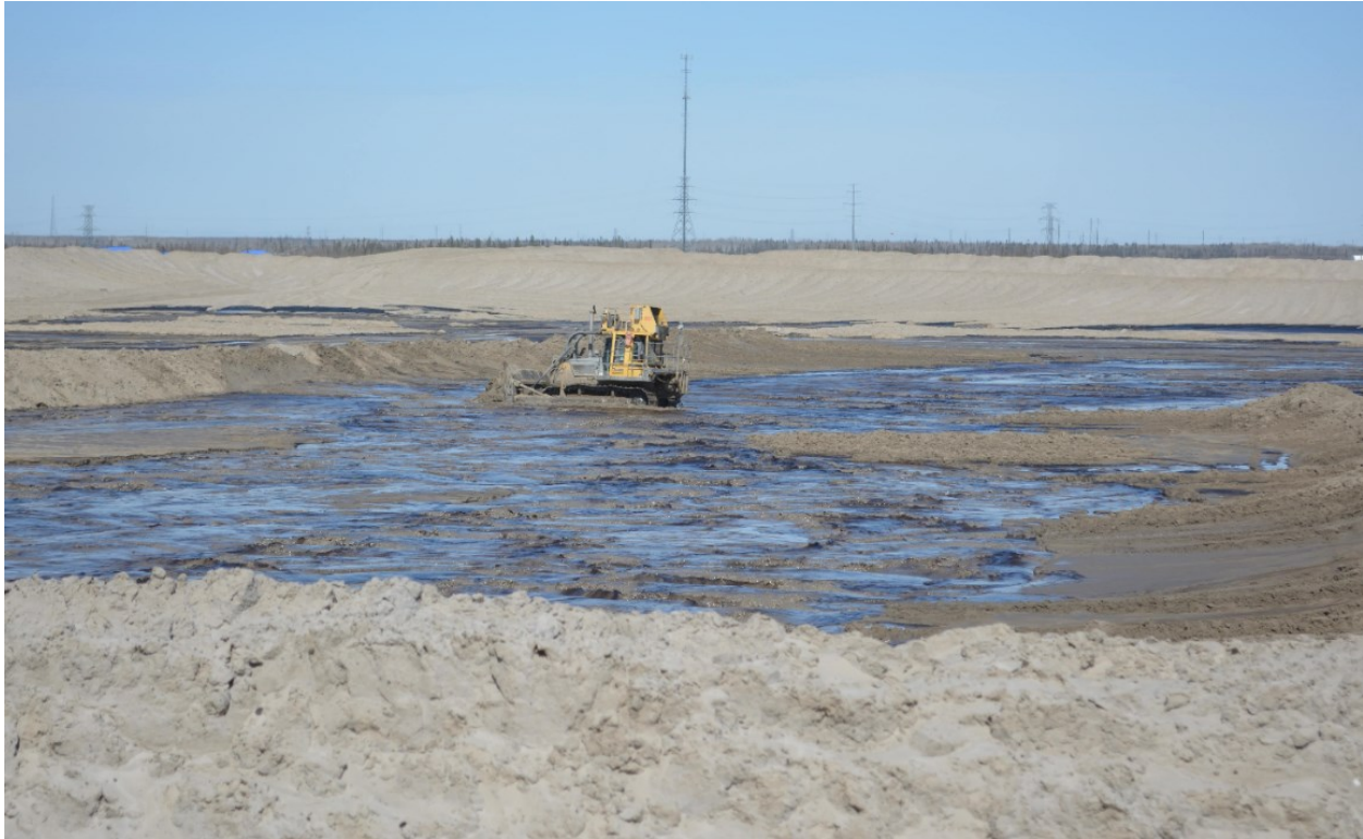
Figure 6. Bulldozer compacting sand in the tailings discharge area.
