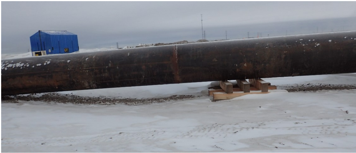
Figure 16. Example of a pipeline elevated on blocking for a full 360° view.
