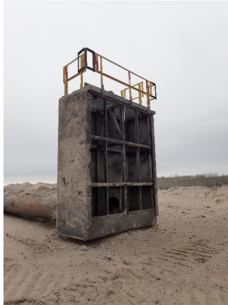
Figure 18. Out of service spill box with handrails installed.
