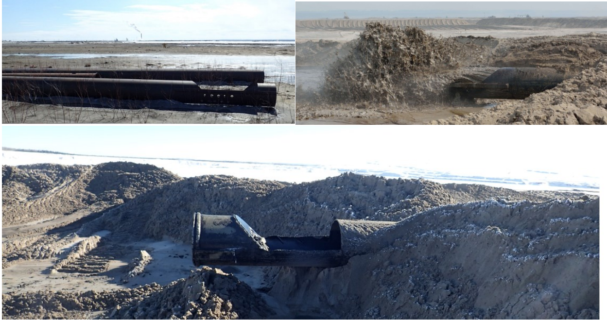
Figure 5. End of line device (or spoon): out of service (top left), in service (top right), and inactive (bottom).
