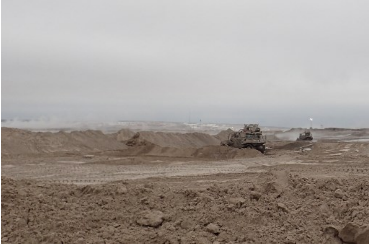
Summer Photo (b), Table 7. Bulldozer creating steep cell walls in tailings discharge area.
