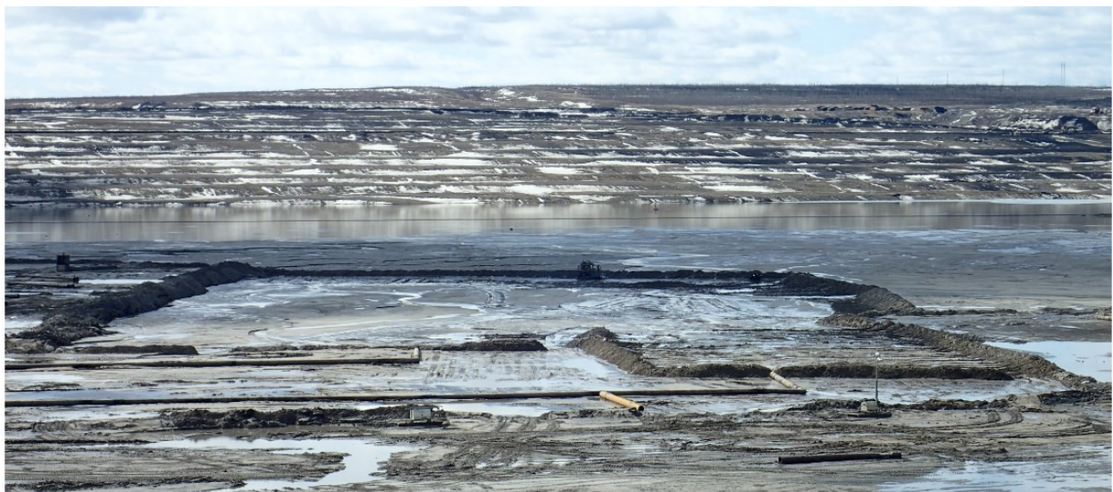
Figure 4. Cell construction in the tailings discharge area at an oil sands mine.
