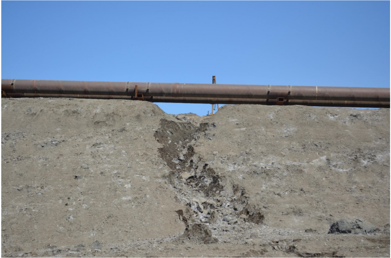
Spring Photo (g), Table 9. Slope in the tailings discharge area with pipeline and erosion features.
