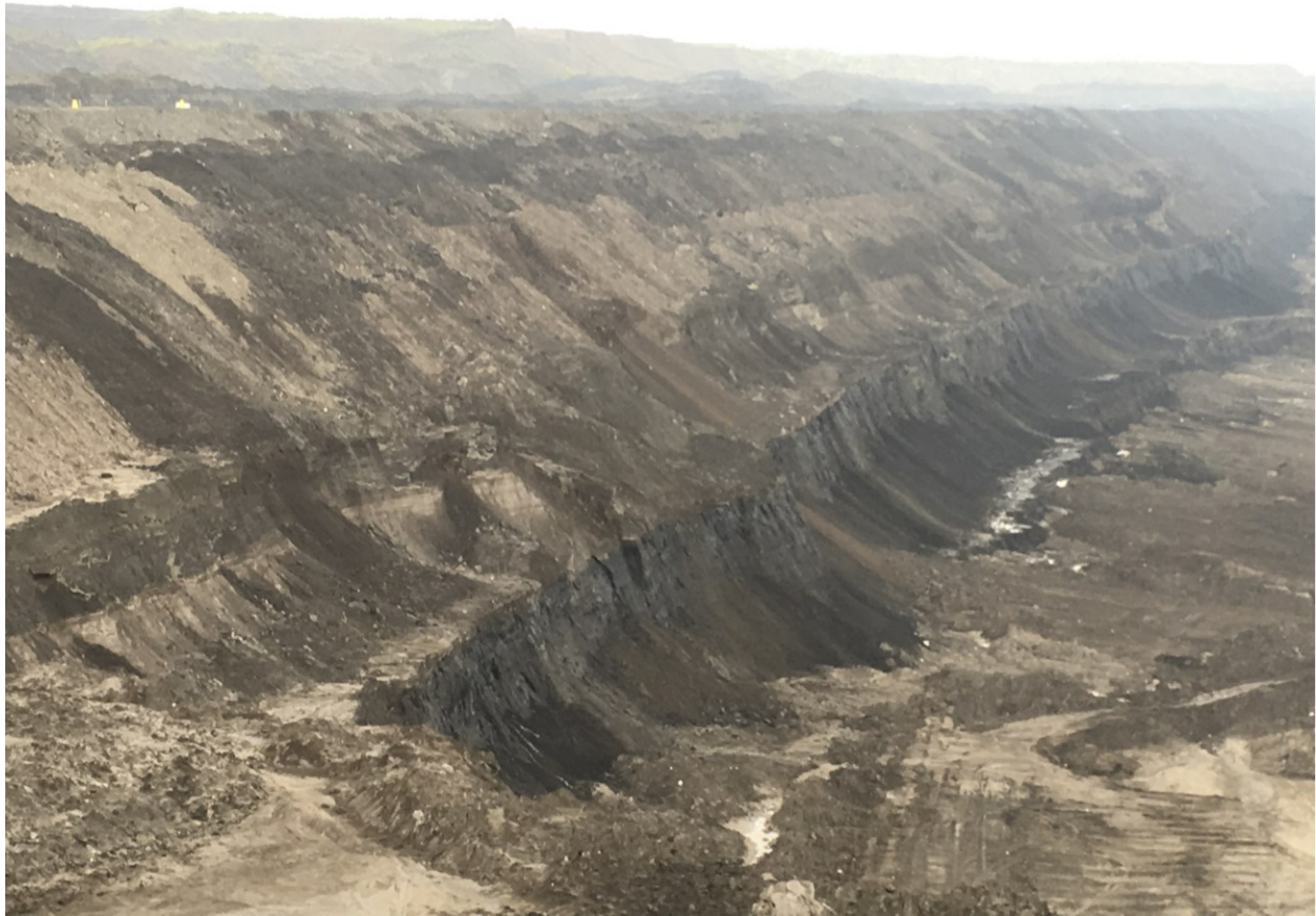
Summer Photo (a), Table 7. View of the open pit (~30 m deep). Steep slopes ( \sim 55^\circ ) typical of mining operations. A failed slope can be seen (top) at an inactive pit area
