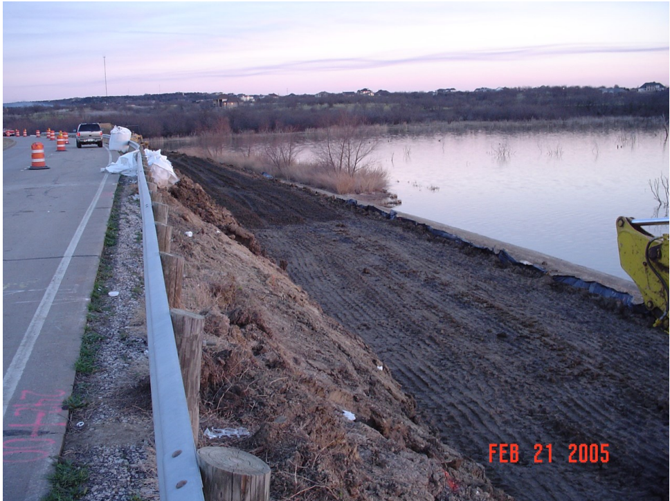
Figure 1.2: Fiber-reinforced soil embankment construction – Lake ridge parkway (Gregory, 2006)
