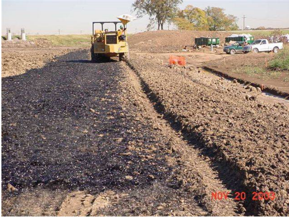
Figure 1.1: Mixing of fiber-reinforced soil on PGBT project (Gregory, 2006)
