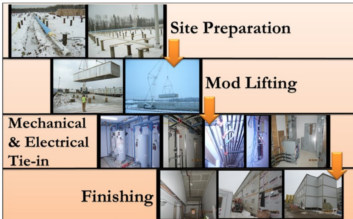
Figure 4-10: Onsite assembly tasks
