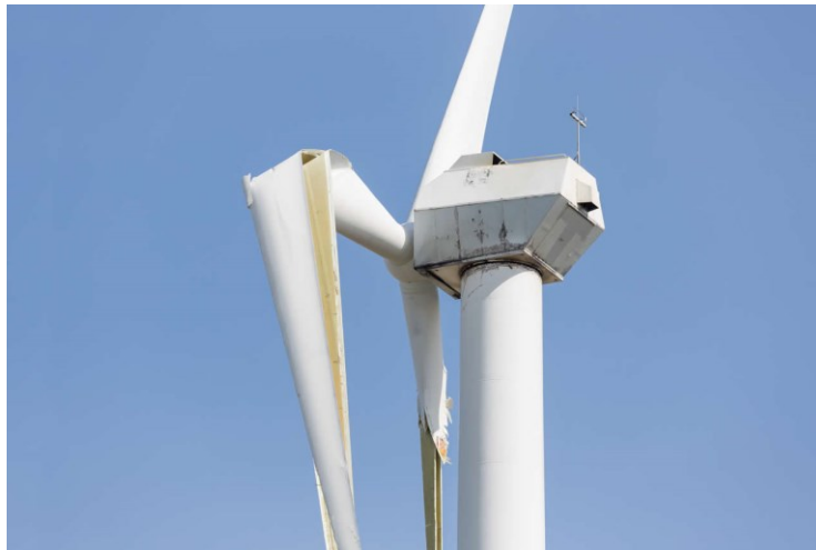
(c) structural collapse [147]
