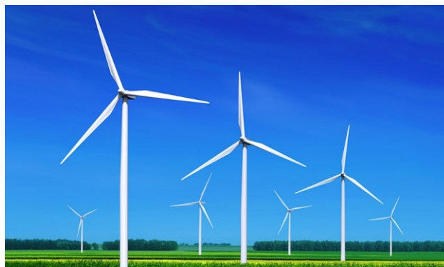
Figure 2-10: Modern onsite horizontal axis wind turbines [48]
