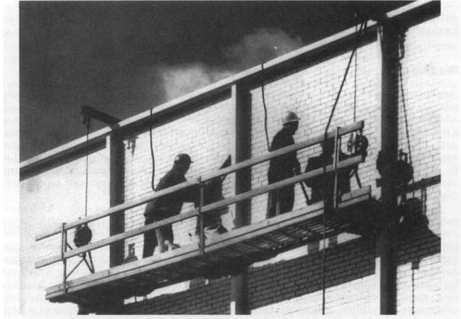
**Figure 2-9 Two point adjustable scaffold**
