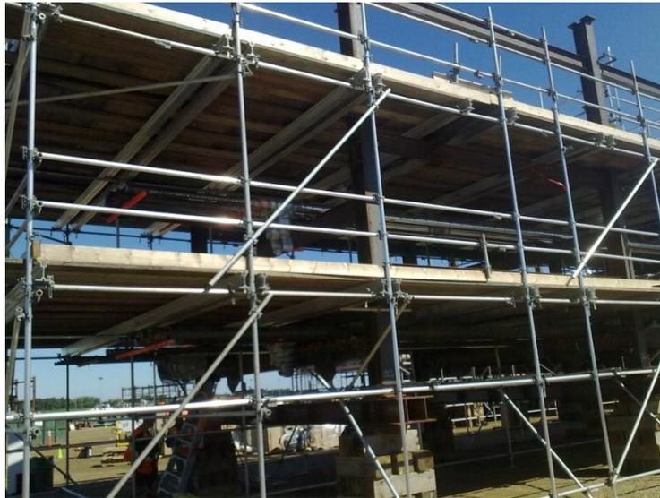
**Figure 2-1 Tube and clamp scaffolding in PCL Modular Yard, Nisku, Edmonton**
