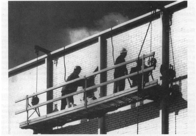
**Figure 2-9 Two point adjustable scaffold**
