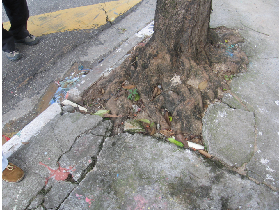
Cracks in asbestos-cement sidewalks from underground tree growth. ©Kyla Elizabeth
