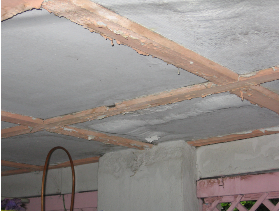
Ceiling containing asbestos materials in state of decay. ©Kyla Elizabeth Sentes, 2006
