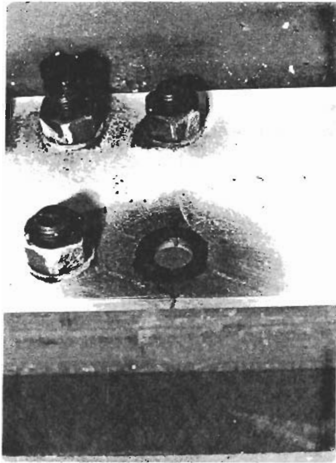
Figure 4.1 Failure Crack in Bolted Test Beam
