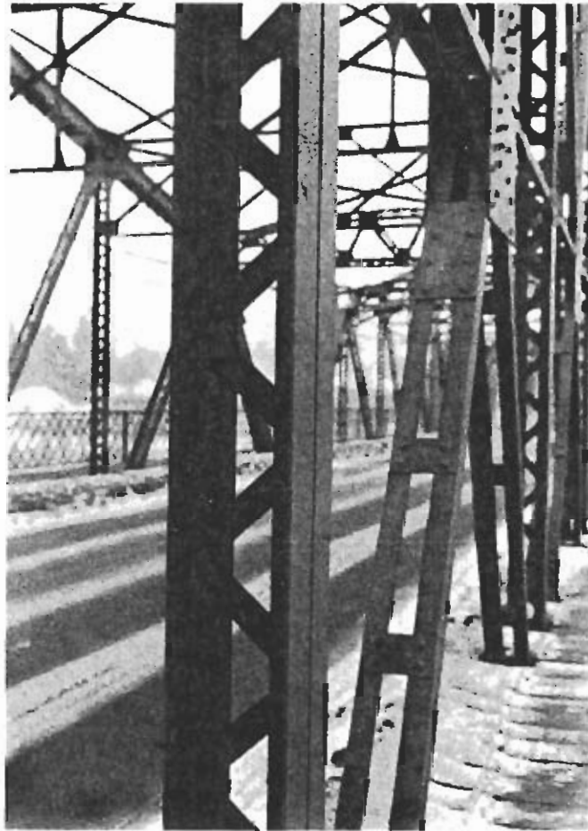
Figure 3.3 Typical Bridge Member
