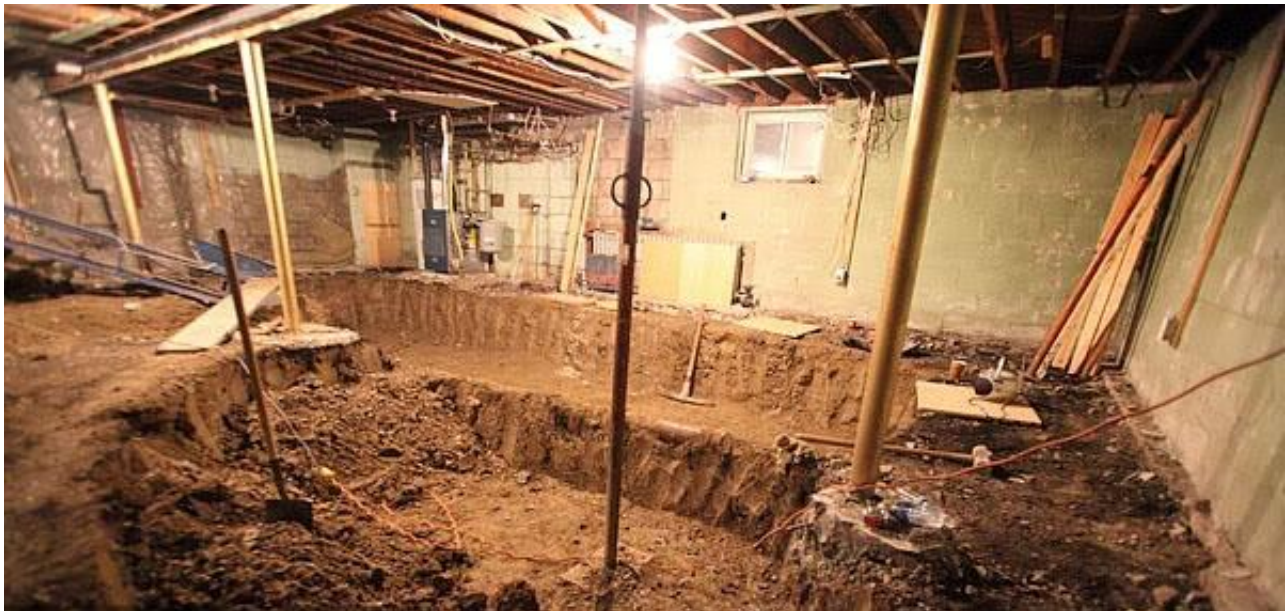
Figure 4-7: Photo of crawlspace during a dug-out basement addition from picswe.com (2018).
