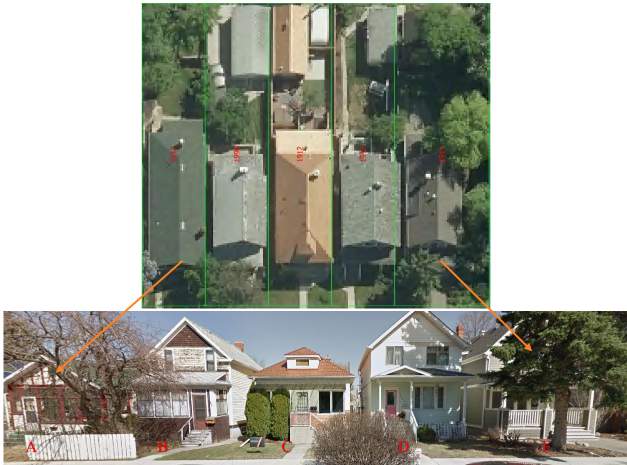
Figure 4-8: [Top] aerial view and [bottom] street view of four pre-war bungalows in Sunnyside [A, C, D, E] (and one home from 1996 [B]). Building D keeps the original pre-war footprint, while A, C, and E have rear oriented main floor additions. Building D and E have second floor additions. Images obtained from Google Maps on 2018-12-01.
