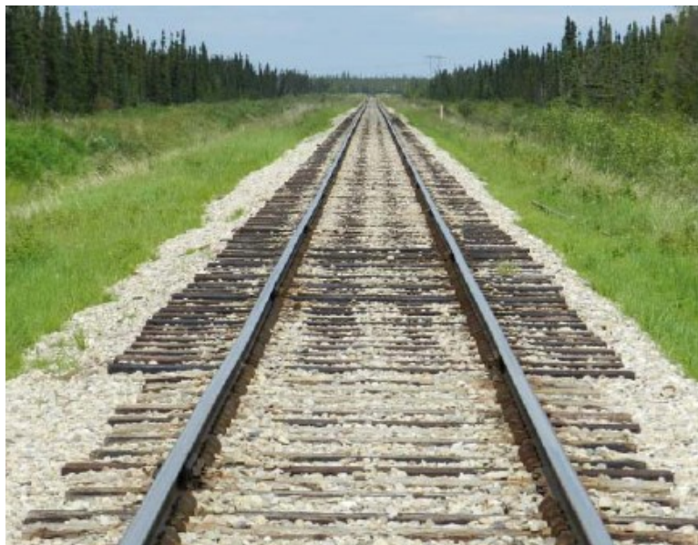
Figure A-2. 3.1 m (10') ties used to improve track performance at muskeg terrain (Bourgonje and Diercks, 2011)
