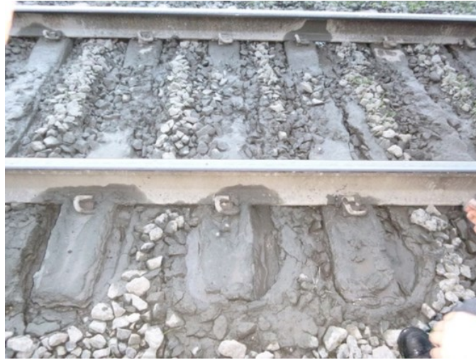
Figure 2-5. An example of mud holes formed in a soft formation near Swan landing on CN's Edson subdivision
