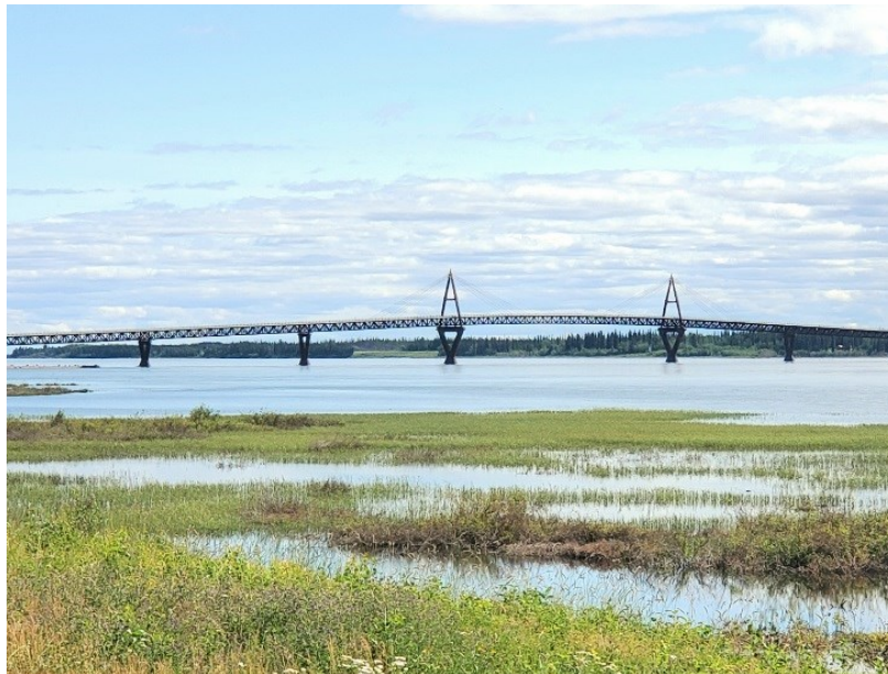
Figure 4: Deh Cho Bridge, Fort Providence, NT
