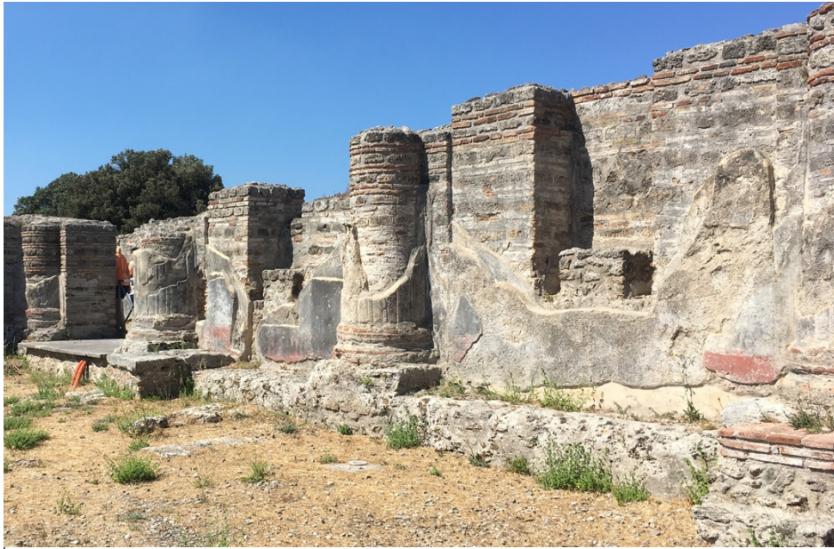
Fig. 11—North wall of Basilica with remains of wall decoration. (Photo: KS Tate)
