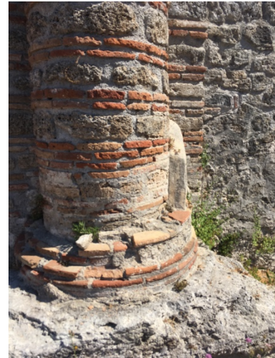
Fig. 10—Detail of brickwork, interior. (Photo: KS Tate)
