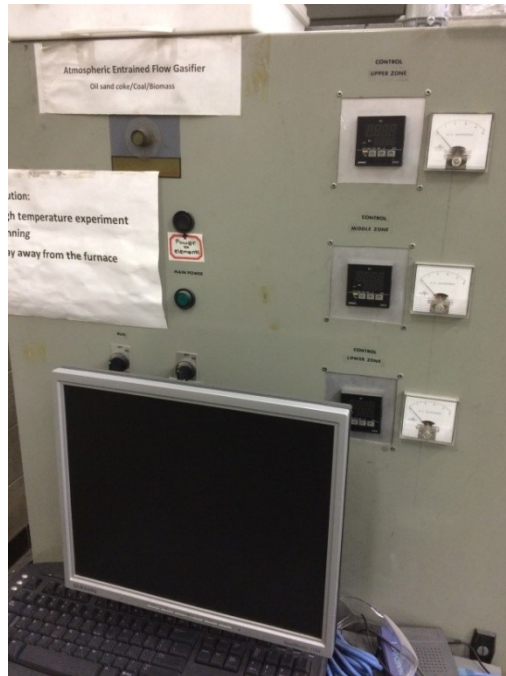
Figure 3: Control board of gasification setup
