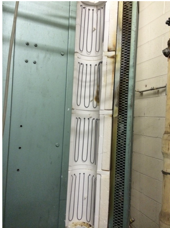
Figure 2: Heating elements of the furnace
