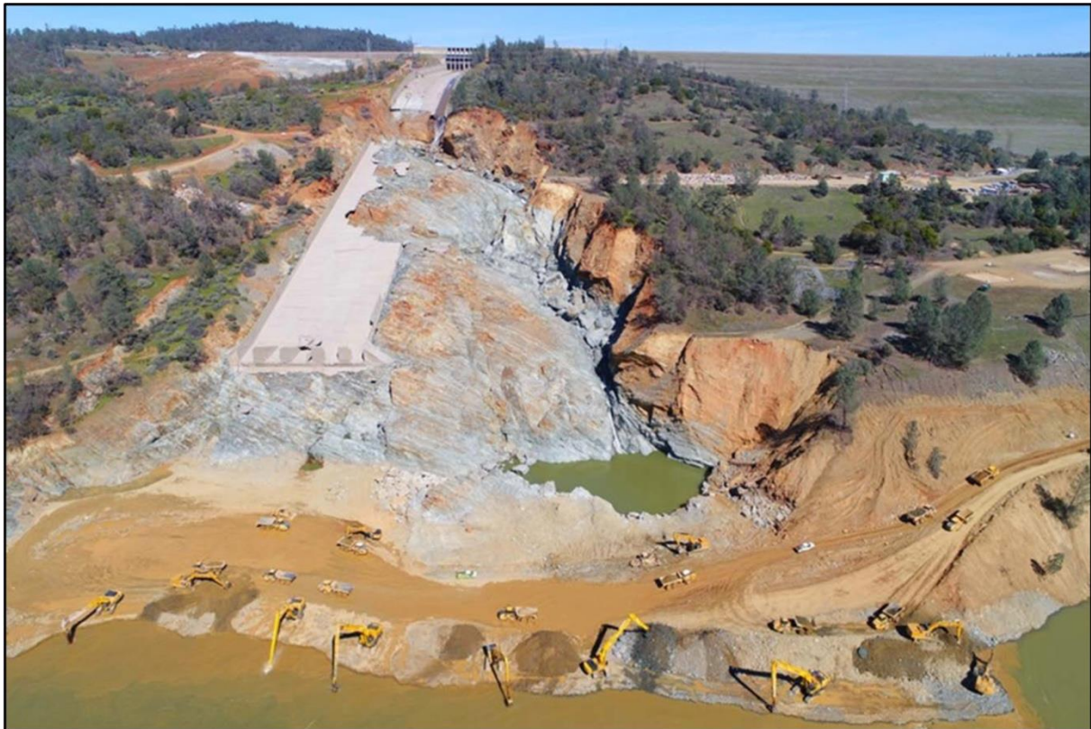
Fig. 6 Oroville Dam Spillway incident (Independent Forensic Team 2018)
