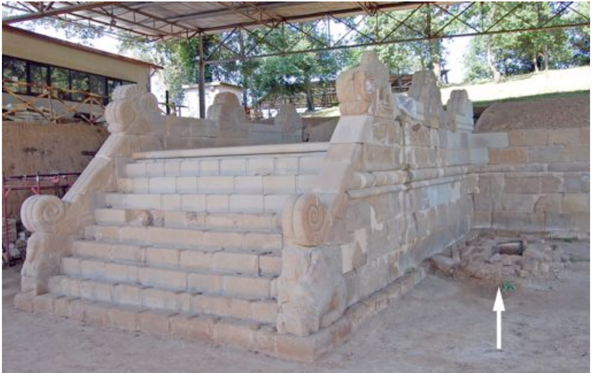
Figure 1.8. The terrace altar, as reconstructed. The remains of Grave S are visible to the right of the altar (arrow). The human remains from this grave were not available for study in May 2010.
